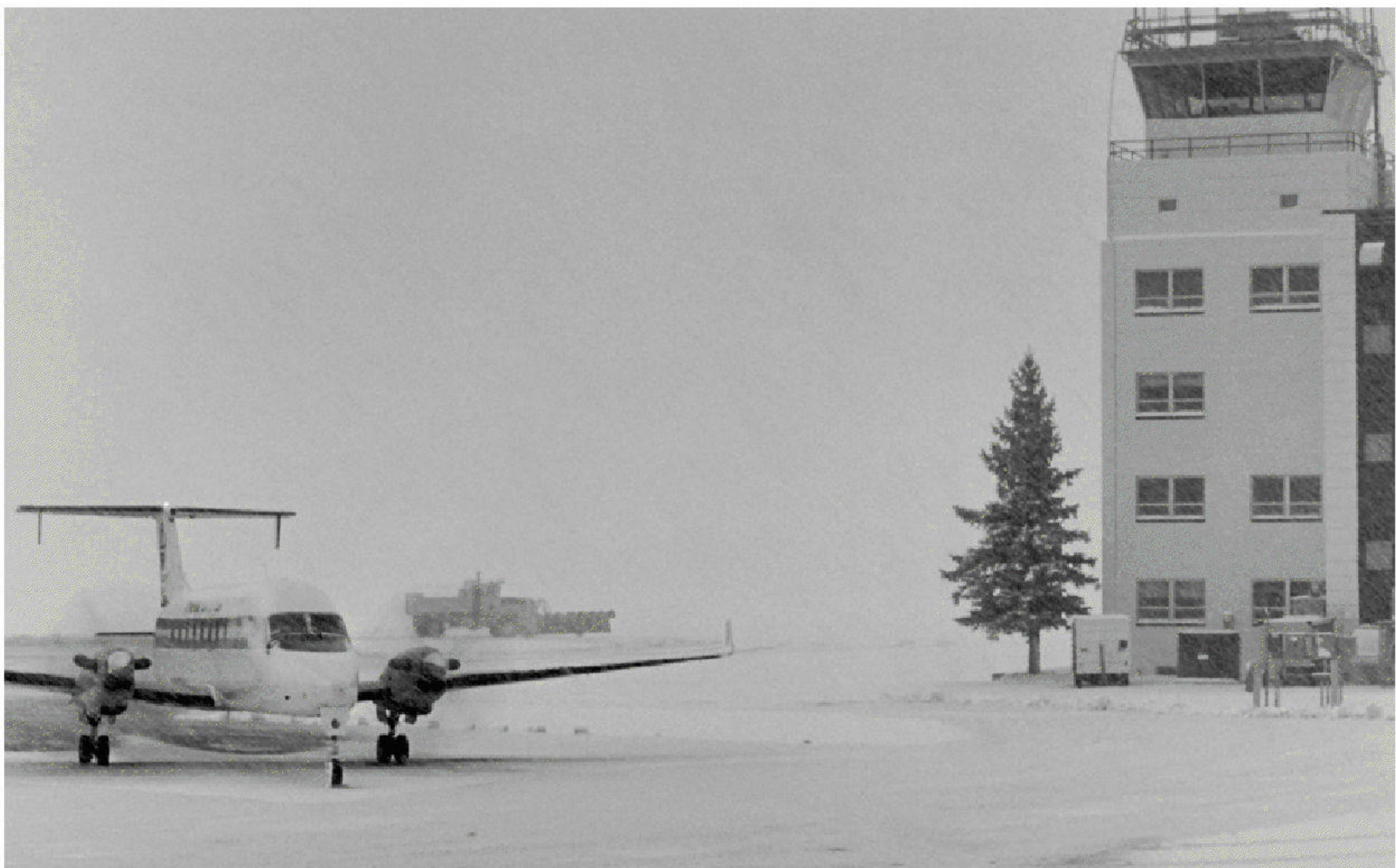
Figure 1-2. Most ATC facilities, such as this control tower at the Cheyenne Regional Airport in Wyoming, are operated by the FAA, although some towers at airports that are not busy enough to qualify for a federal tower are operated by private corporations under contract to local governments. More privatization of the ATC function is possible, as lawmakers search for ways to reduce federal spending.
