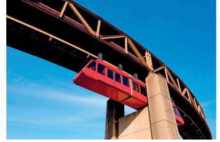
Photo 1.2 This bridge truss consists of two-force members that may be in tension or in compression. ©Natalia Bratslavsky/Shutterstock
